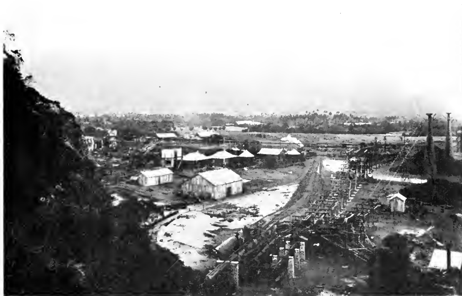
Smelter Yard at Thio.
